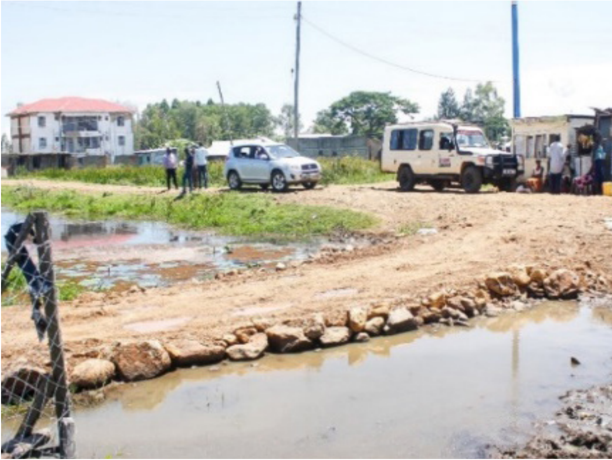
A community improvised dyke in a flooded area at Kapuodhe, along the Nyamasaria river and dyke
