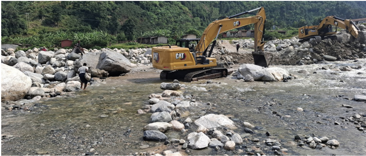
Heavy machinery employed by government to desilt the river-bed
