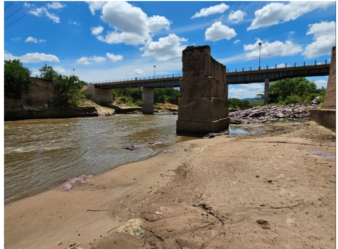
Figure 17: Mara River across new Nyansurura Bridge on the Tarime Road; Fore front are the remains of the old bridge that was destroyed by floods.
